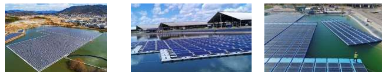
Figure 9 : Centrales photovoltaïques flottantes
